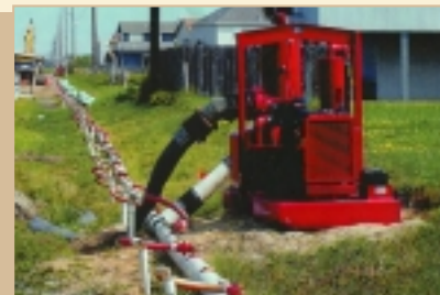
Wellpoint system, Galveston Texas.
